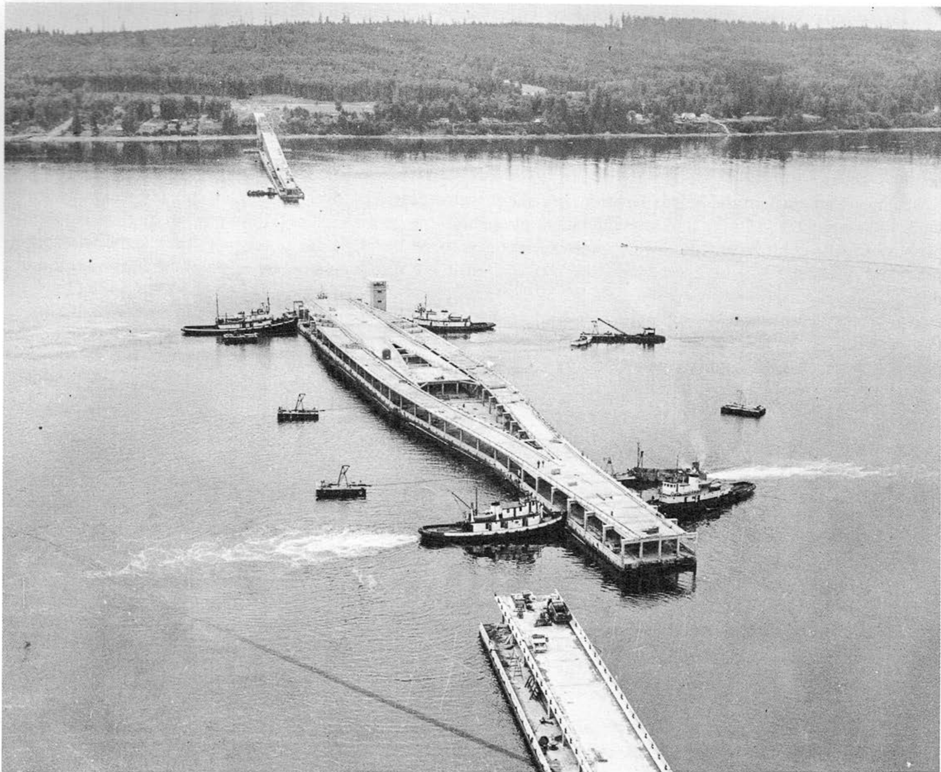
Five Foss tugs, LESLIE, EDITH (3), WEDELL, ANDREW and CAROL (just visible) positioning one of the center spans of the Hood Canal Bridge in 1960. (Courtesy of Foss Tug Co)
